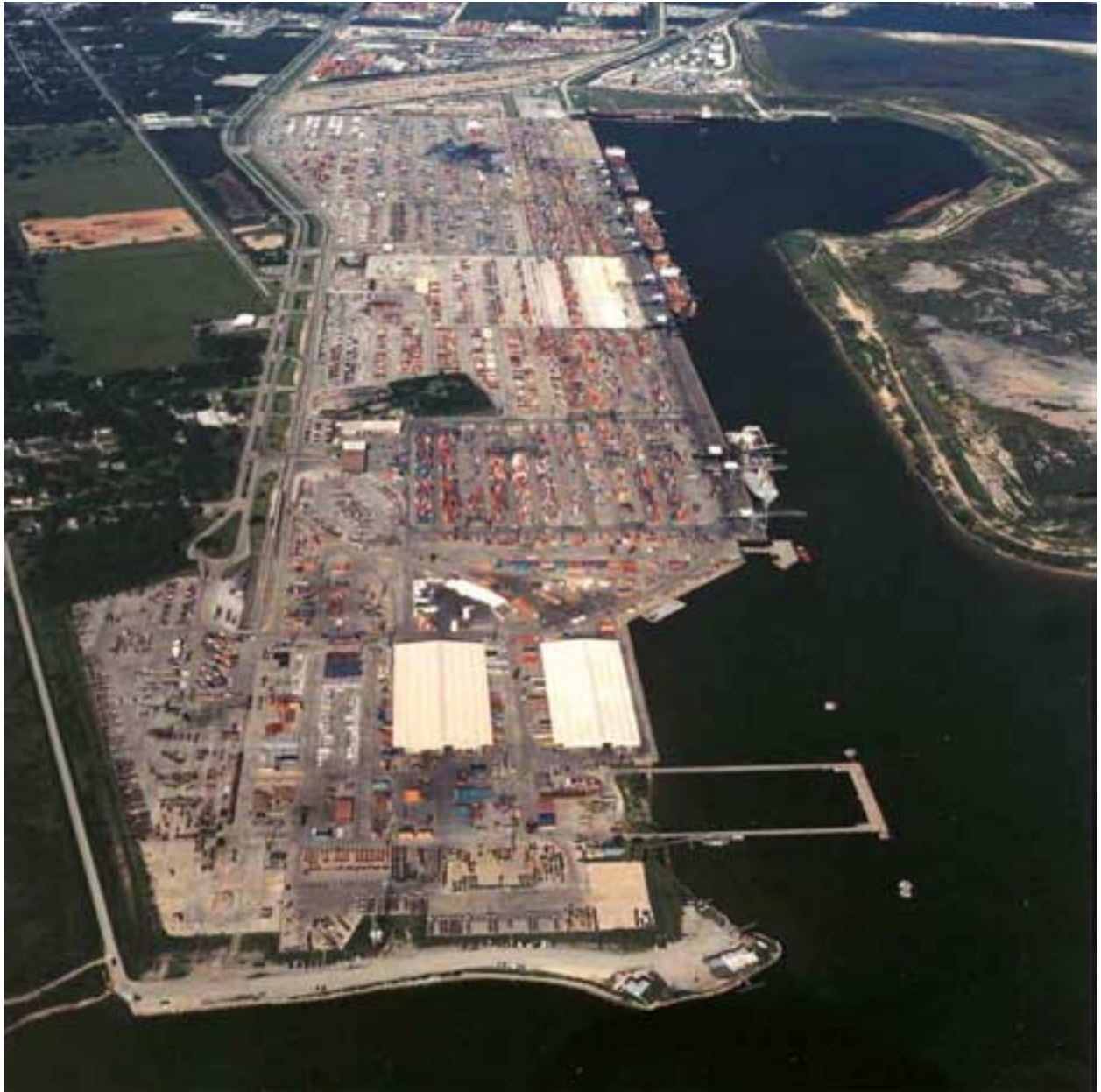
Figure 1 Barbours Cut Terminal
